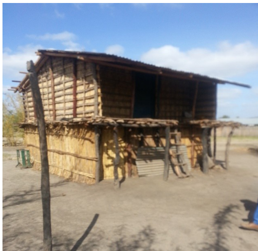
Figure 1. Adaptation of residential houses in the flood prone areas in the study area, as a strategy to avoid relocation and loss of proximity to livelihood-essential resources.
