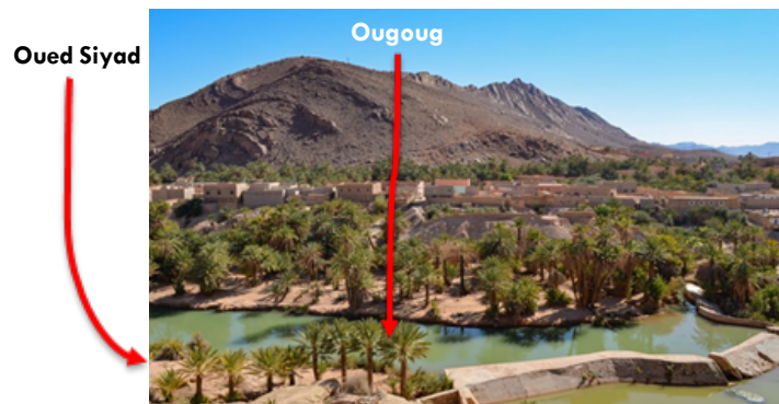
Figure 4. The Diversion Dam at Taghijit Oasis Source: Cliché Personal 2019
