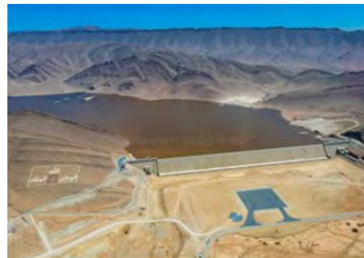
Figure 6. Location of the Fask Dam Source: Noufel El Majdoubi, 2024
